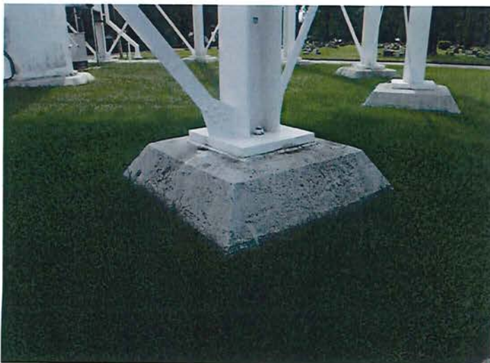
6) Typical leg foundation is in good condition.
