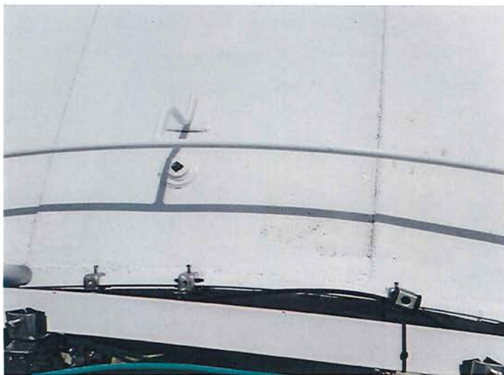
39) The painter's railing is in good condition.
