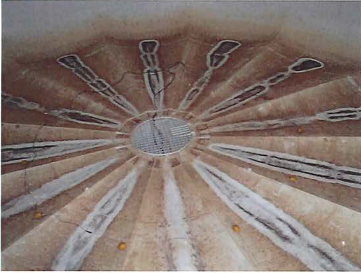
52) The bowl coating is in good condition.
