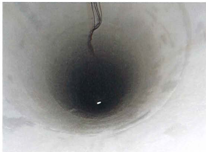
54) The riser coating is in good condition.
