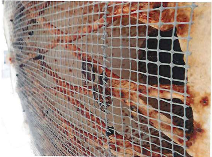
11) The overflow pipe screen is in fair condition.
