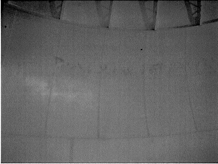
49) The sidewall coating is in good condition.
