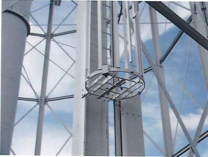
13) There is a vandal guard on the leg ladder.
