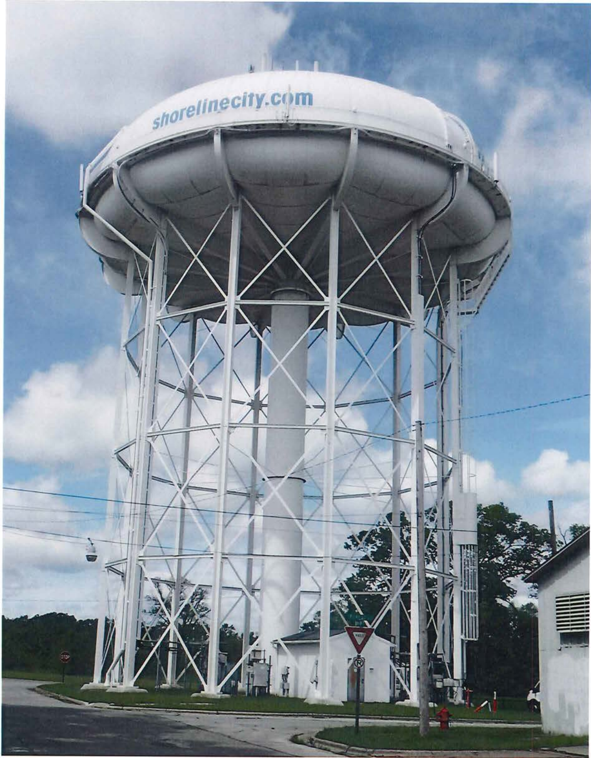
1,000,000 gallon radial arm tank (Nims) located in Muskegon, Michigan.
