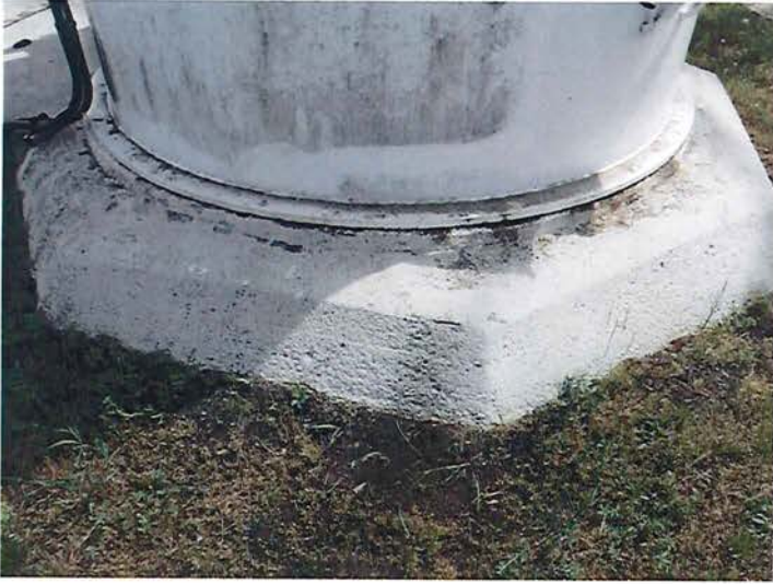
1) The riser foundation is in good condition.
