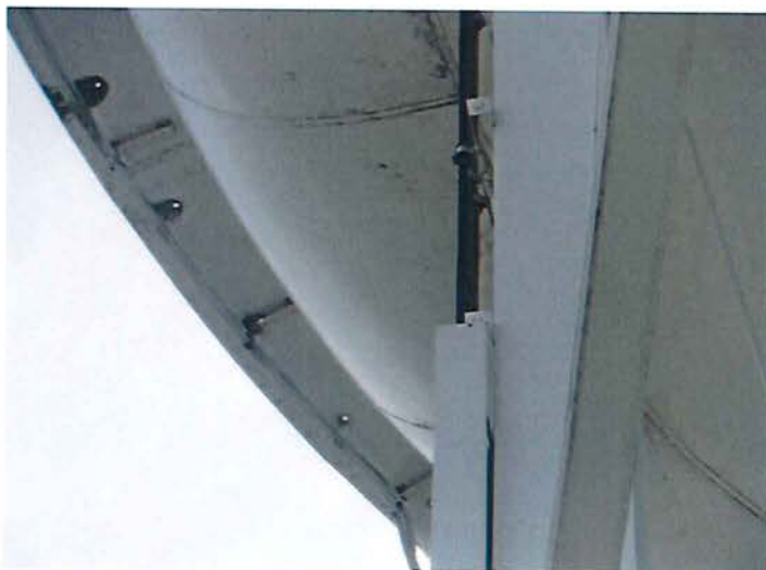
18) Antenna cable routing up a leg with a shroud.
