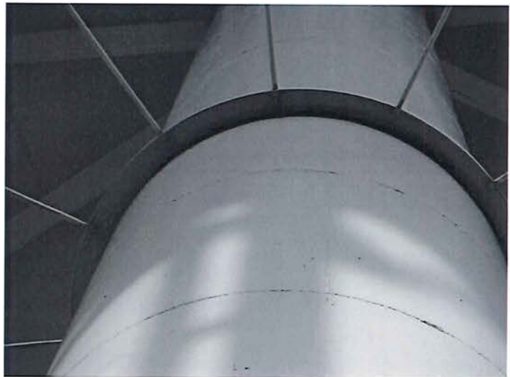
5) The riser rod connections are in good condition.
