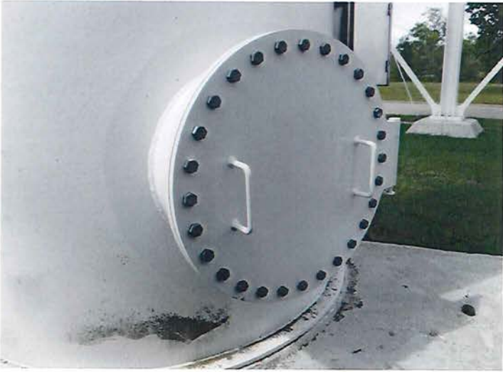
3) The 30 inch riser manway is in good condition.
