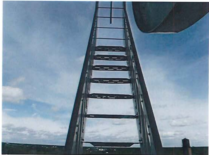
23) Stairs and ladder rungs up to the balcony.
