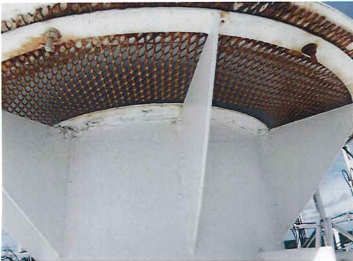
42) There are gaps in the vent screen around the outer edge and the screen is oversized.
