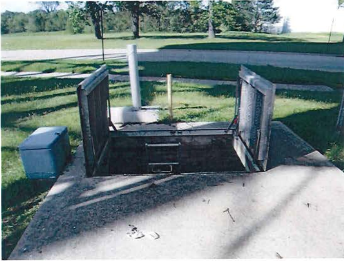
58) Hatch to the pit next to the tank.
