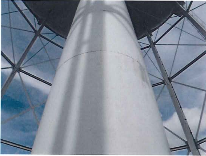
4) The riser coating is in good condition.
