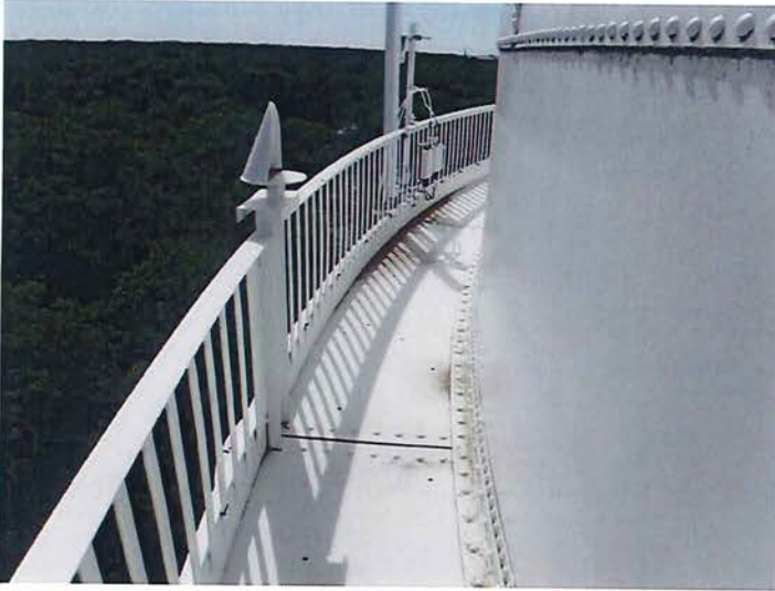
25) The balcony coating is in good condition overall.
