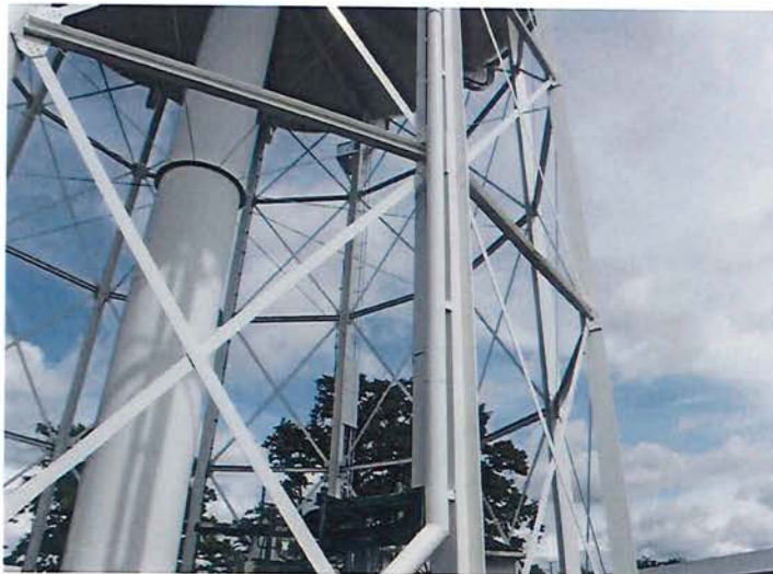
15) The coating is in good condition on the legs.
