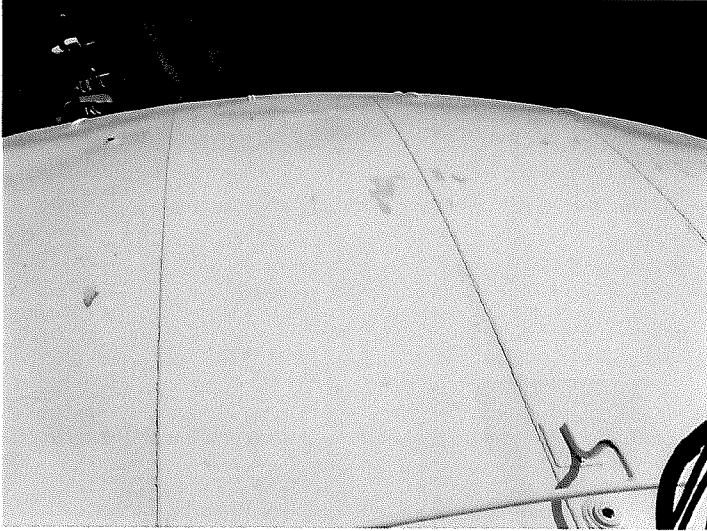
34) The roof coating outside the handrail is in good condition overall.
