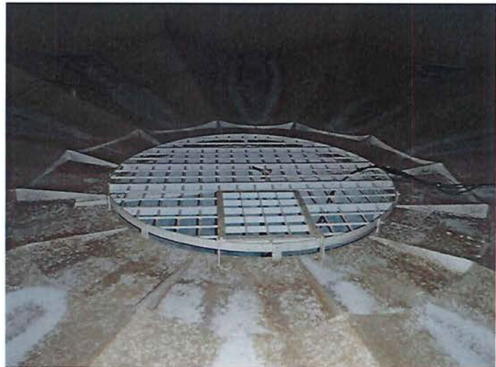
53) The riser grate is in good condition.
