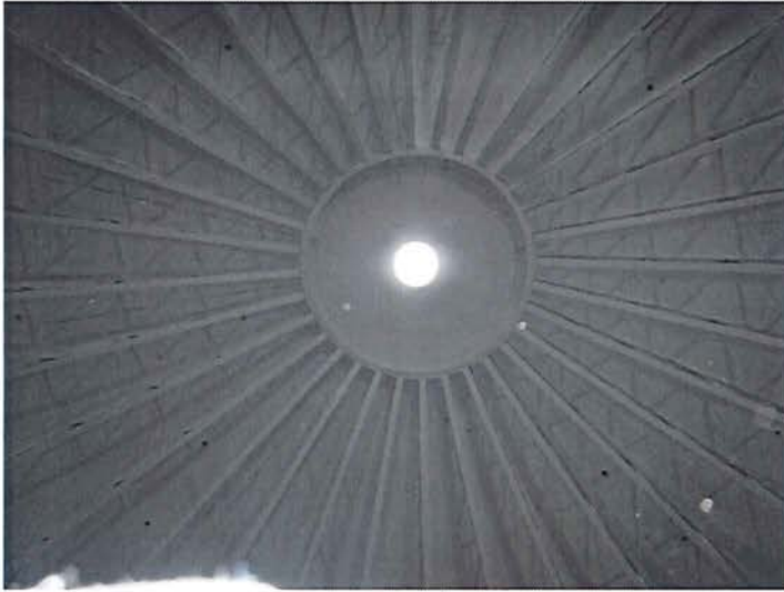
43) The wet interior roof coating is in good condition.
