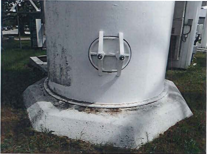
2) The original riser manway is in good condition.
