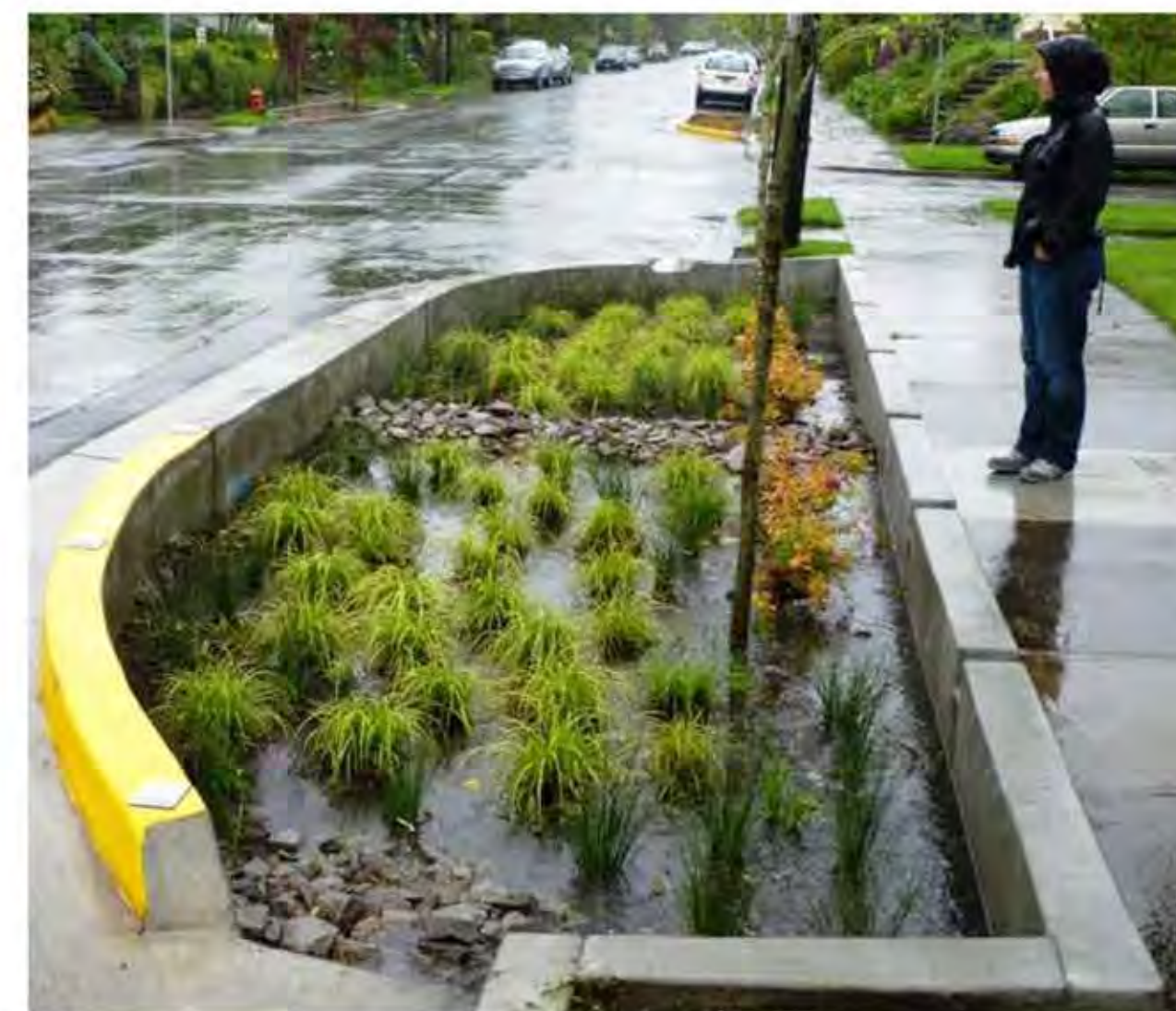
3 BIOSWALE SCALE: NTS
