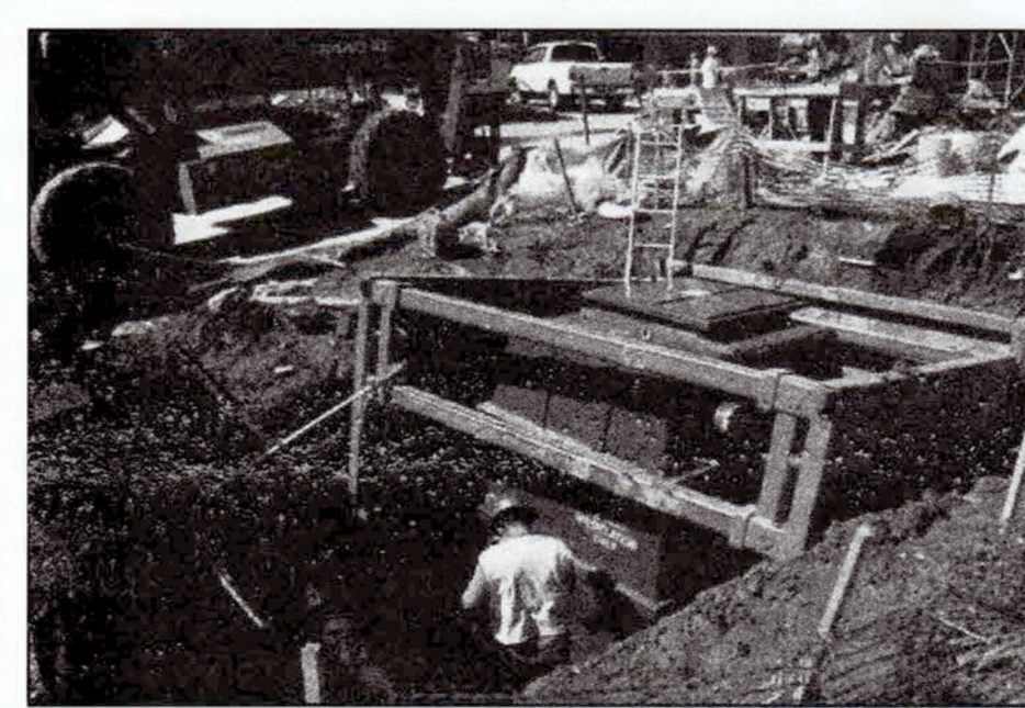
VAULT IN POSITION PROTECTED BY 'CAVE-IN' BARRIER
