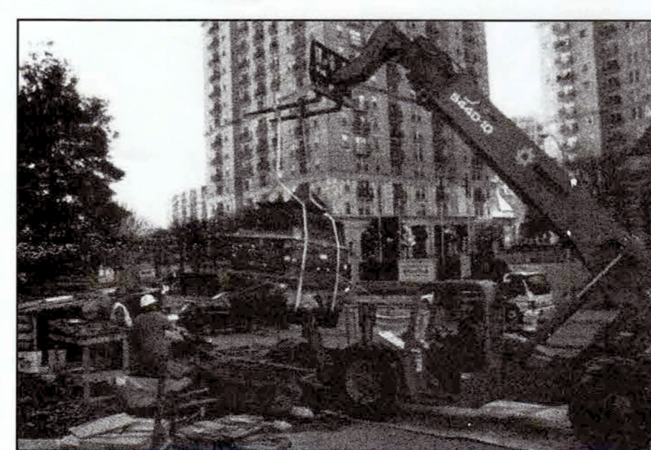
LIFTING FORK CRANE WITH DOUBLE STRAP SLING
