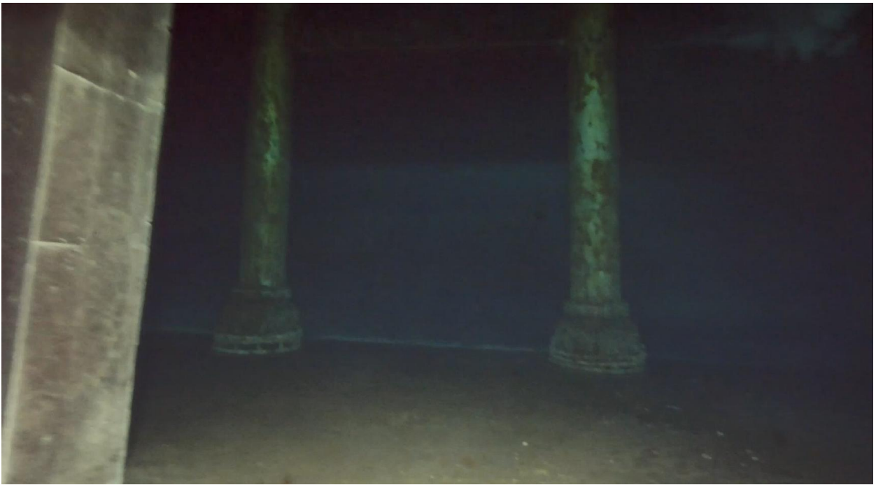
BACKWASH PUMP SUCTION LINES & FOOT VALVES
