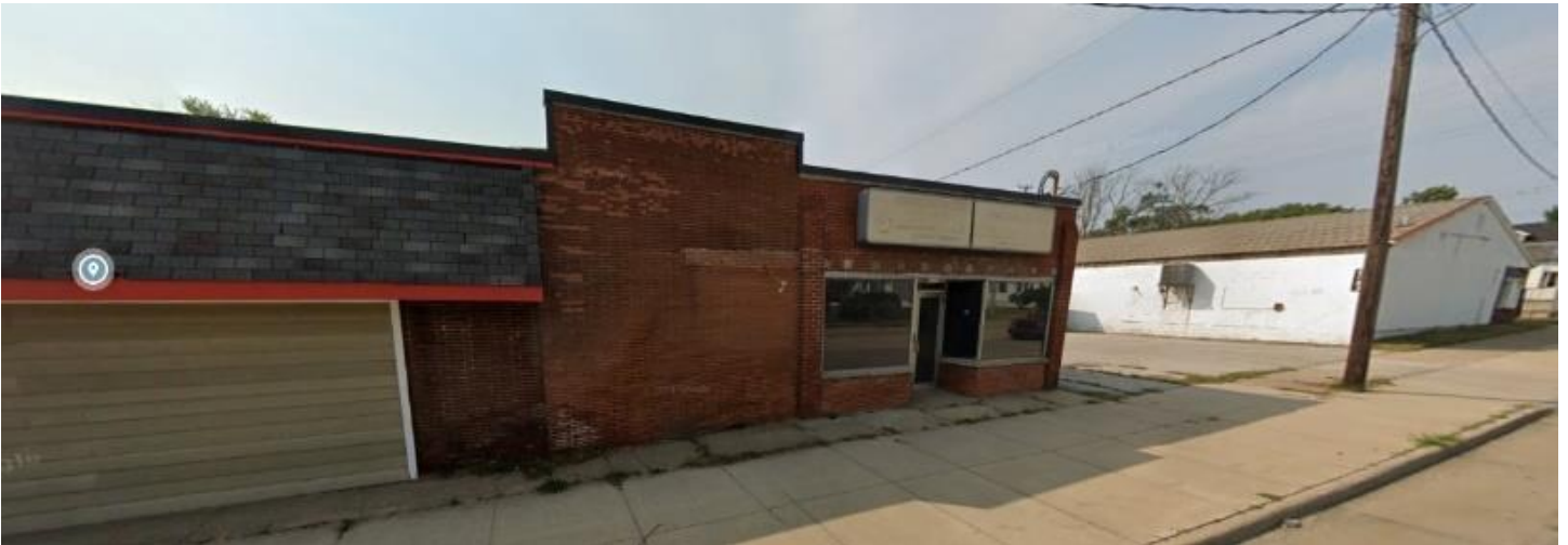
Uninteresting/blank walls on industrial/commercial properties make for a bland commercial district.
