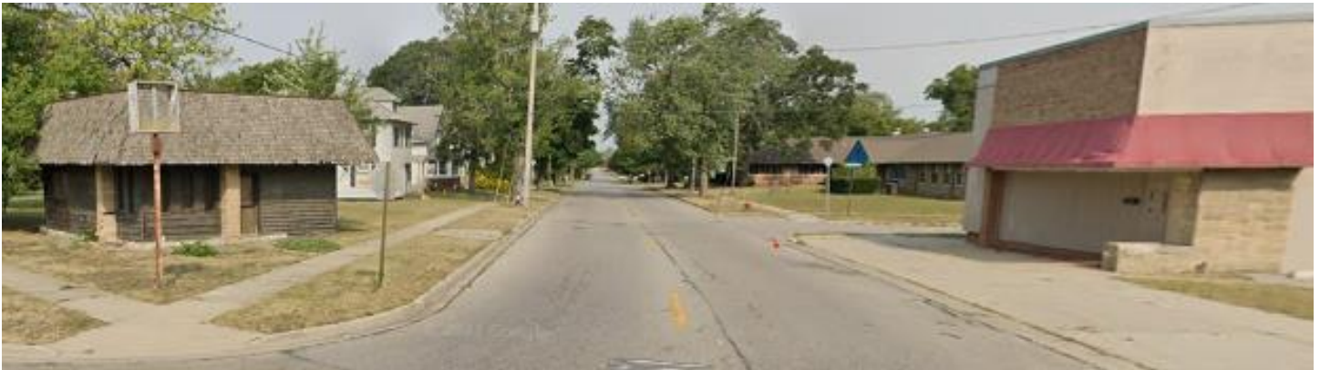
The underutilized business corridor at Terrace Street and Irwin Avenue is plagued by vacant and deteriorating buildings.
