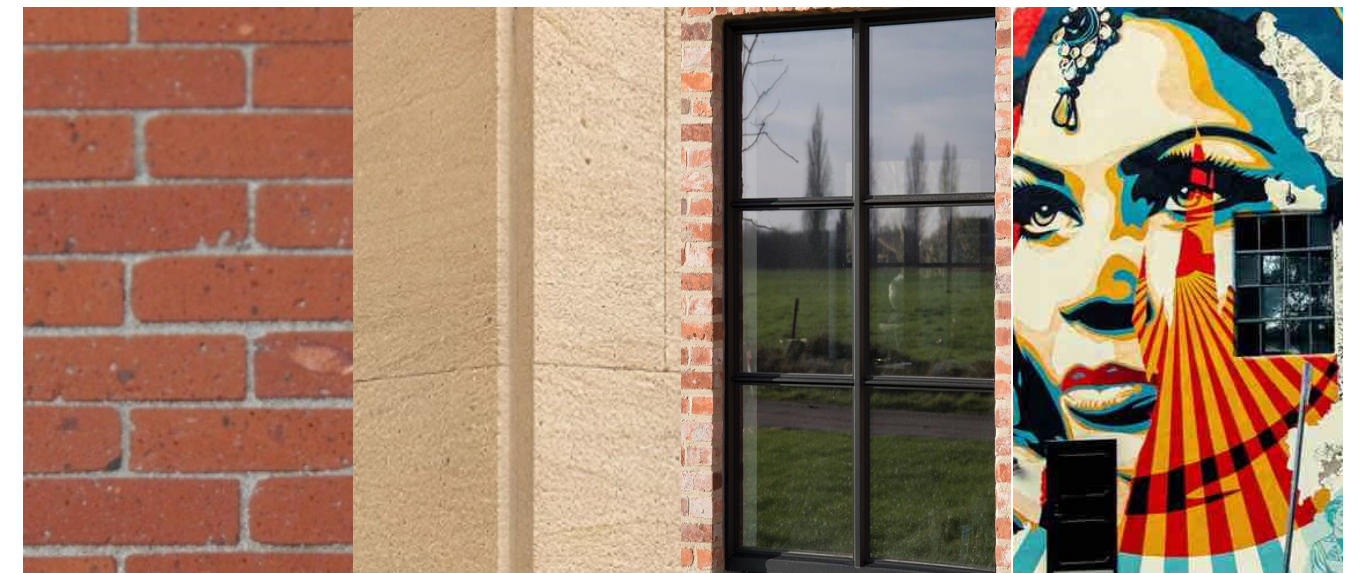
Figure 78: Comparison of a Building's Façade Before and After Implementing Improvements
