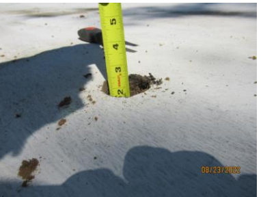
METAL DECK 1.5" PERLITE MOD BIT COATING
