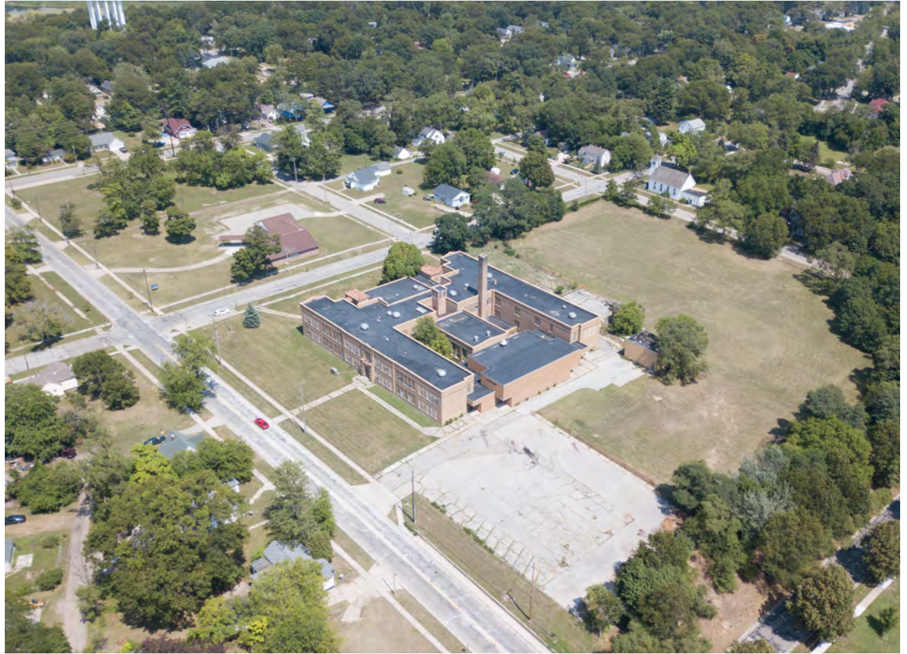
Froebel School building and surrounding land
